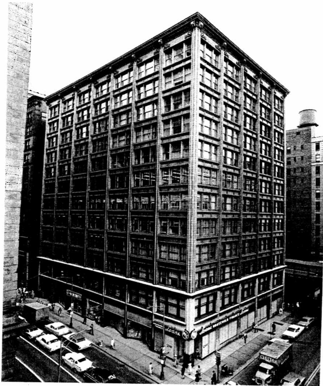
This Richard Nickel photograph of the Brooks Building dates from the 1960s. The building is little changed from its original appearance (see photo on inside front cover), retaining both its original cornice and much of the character of its lower two floors, which are clad in marble.
